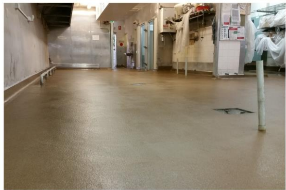
*The transformation of a severely damaged kitchen
